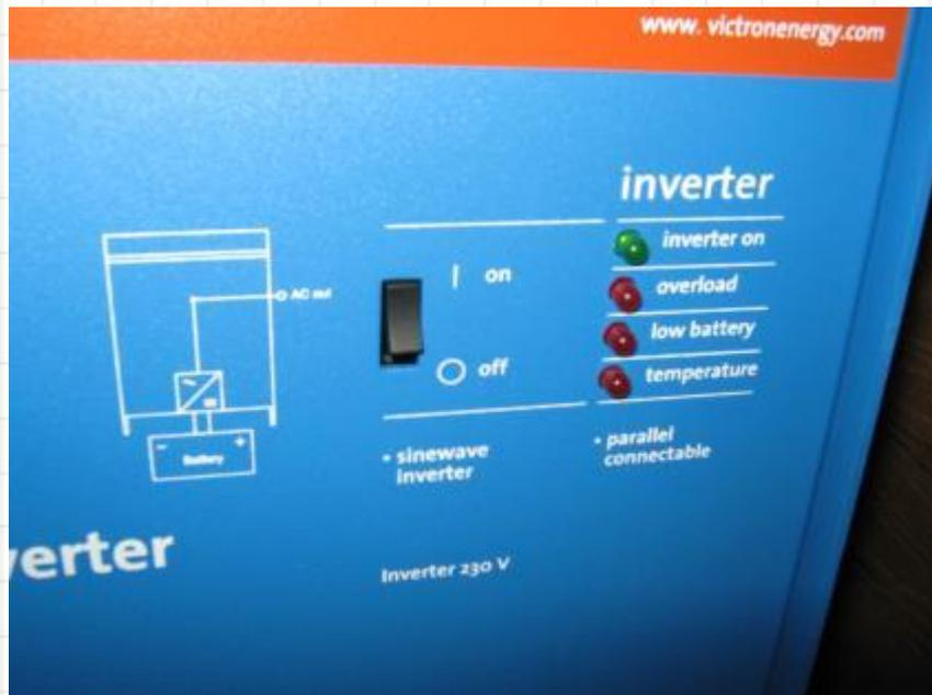
The switch should be left in the ON position at all times.
